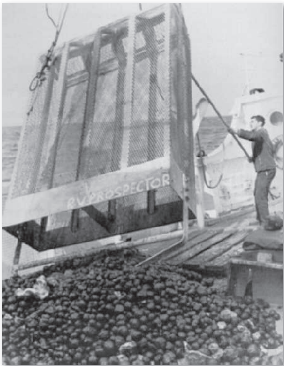
Figure 4.29 Mining manganese nodules. Manganese nodules can be collected by dredging the ocean floor. This metal dredge is shown unloading nodules onto the deck of a ship.
