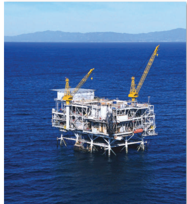
Figure 4.25 Offshore oil-drilling platform. Constructed on tall stilts, drilling platforms are important for extracting petroleum reserves from beneath the continental shelves.
